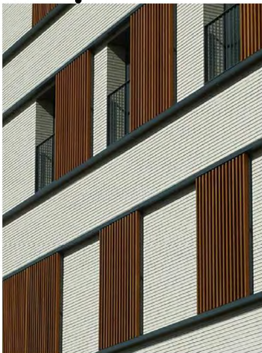
TIMBER SCREEN DETAIL
